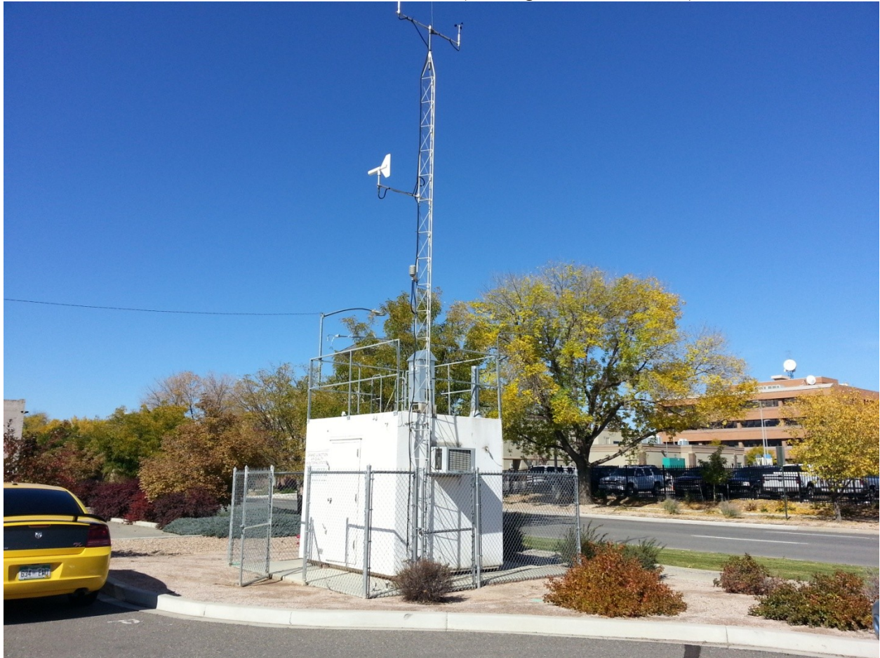
Site Photo: Shelter and inlets (looking NORTHWEST )
